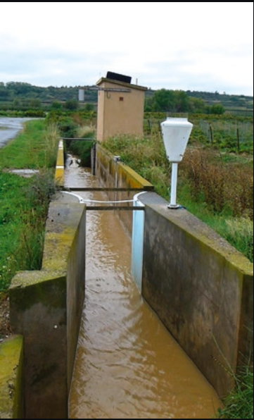
▲ System for measuring water and rainfall flows and quality at the outlet of the site
